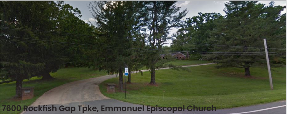
7600 Rockfish Gap Tpke, Emmanuel Episcopal Church A historic, red brick, picturesque church rebuilt 1911-14 in the Colonial Revival style, sublimated within landscape
